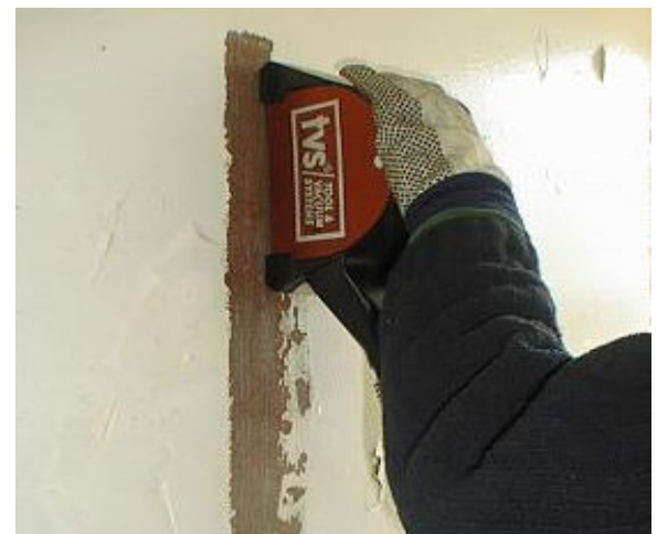
Removing coatings to a bare metal finish
